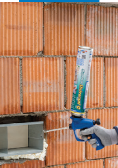
Filling a ventilation channel
