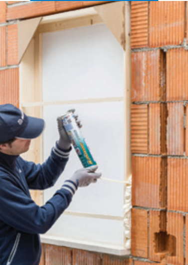
Filling gaps between a window frame and wall
