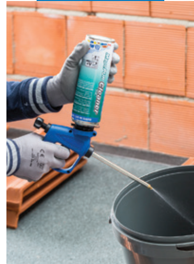
Cleaning a foam filler extrusion gun
