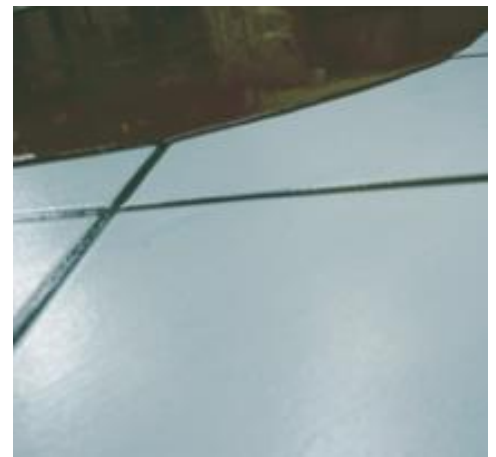
Application of Ultraplan with a metal trowel on an existing ceramic tile floor after the application of Eco Prim T Plus
