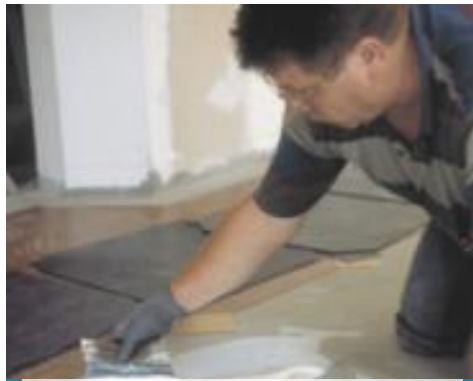
An example of an installation of inlaid PVC on a surface levelled with Ultraplan - CD2 - Milan - Italy
