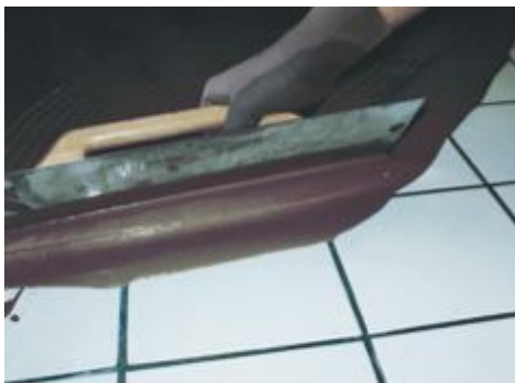
Application of Ultraplan with a metal trowel on an existing ceramic tile floor after the application of Eco Prim T Plus
