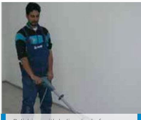
Polishing with helicopter before applying Ultraplan Eco - Mirabello kindergarten - Cantù (Como) - Italy
