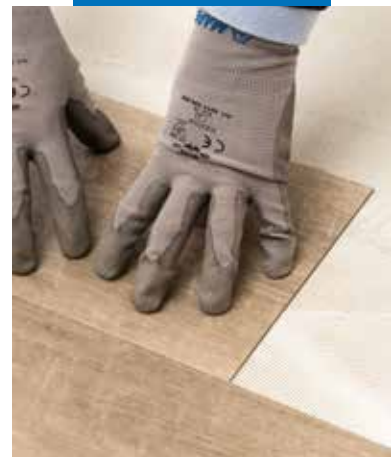
Installation of LVT with Ultrabond Eco V4 Evolution
