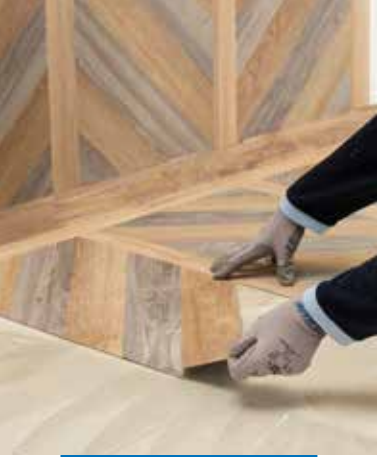
Installation of MODULAR LVT with Ultrabond Eco V4 Evolution
