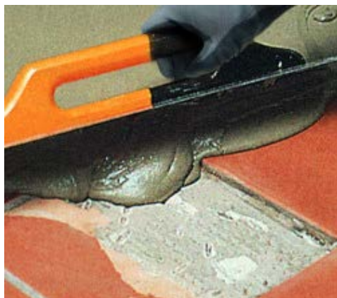
Filling holes with Nivorapid
