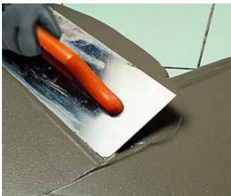
Levelling of existing floor with Nivorapid
