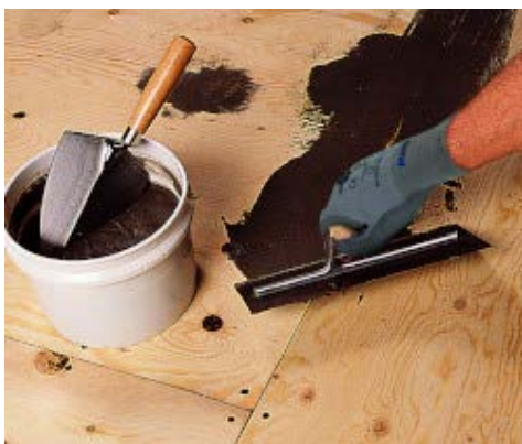
Grouting a plywood substrate with Nivorapid + Latex Plus
