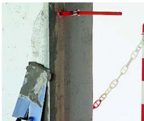
Repairing vertical surface with Nivorapid
