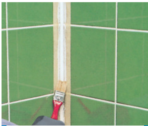
Smoothing the joint with soapy water and a small brush
