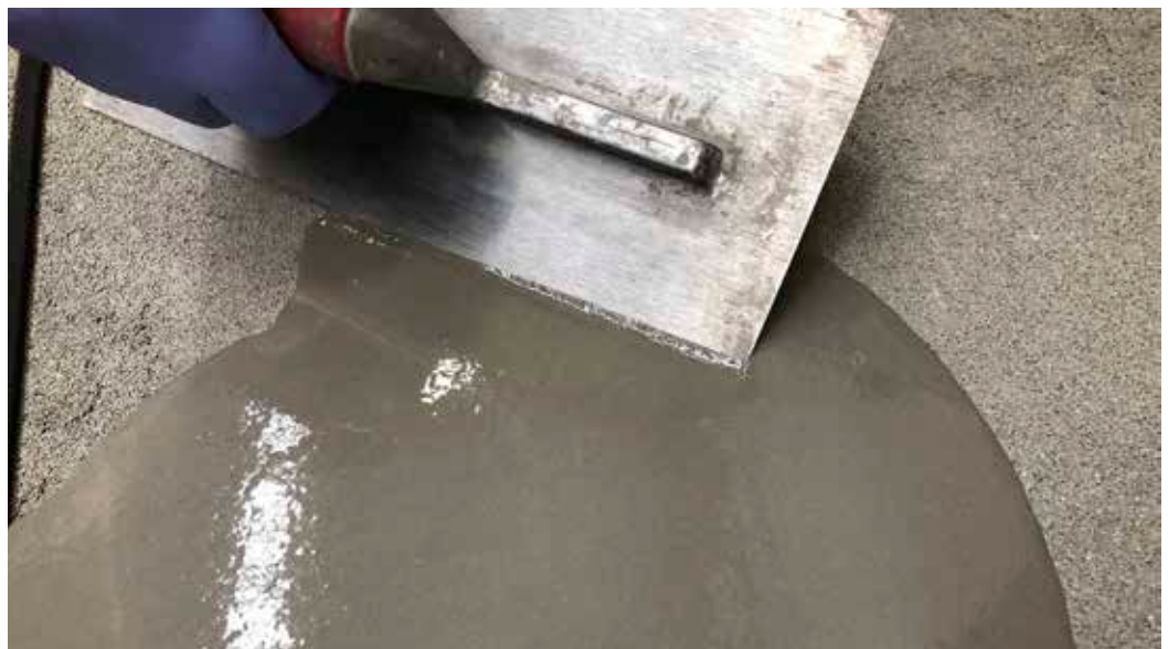
Installation of Ultraplan Trade after first priming the porous concrete substrate using Eco Prim T Plus diluted 1:2 with water
