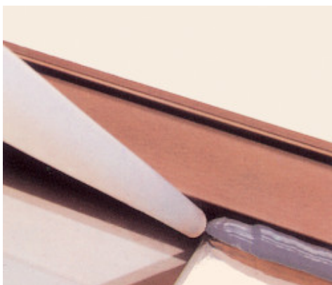
Sealing aluminium window frame with Mapesil AC
