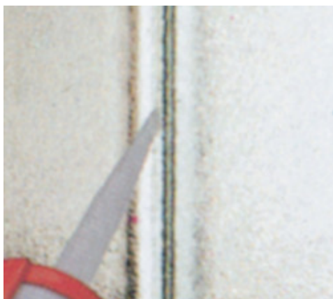
Sealing U-profile glass
