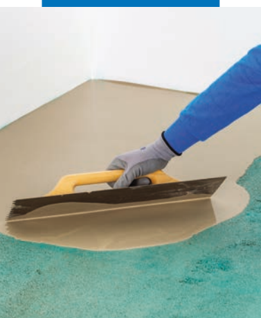
Self-levelling compound application on Mapeproof Primer
