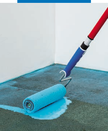
Second coat application of Mapeproof Primer
