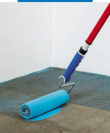
First coat application of Mapeproof Primer
