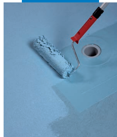
Application by roller of Mapelastc AquaDefense second coat
