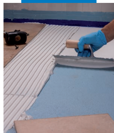
Bonding tiles on Mapelastc AquaDefense
