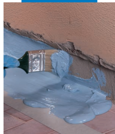
Application of Mapelastc AquaDefense by brush between floor and wall before applying Mapeband
