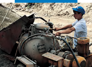
Mixing Mapecem with an automatic pumping unit
