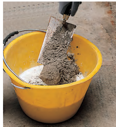
Mixing Mapecem with Planicrete SP to make a bonding slurry
