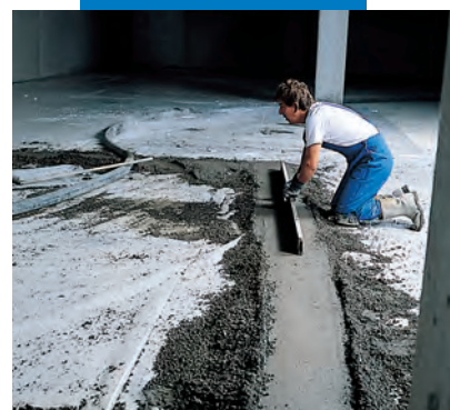
Preparing a levelling strip
