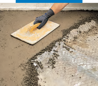
Covering pipes with Mapecem and reinforcement netting
