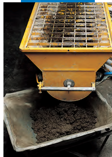
Mixing Mapecem in a mini-batcher
