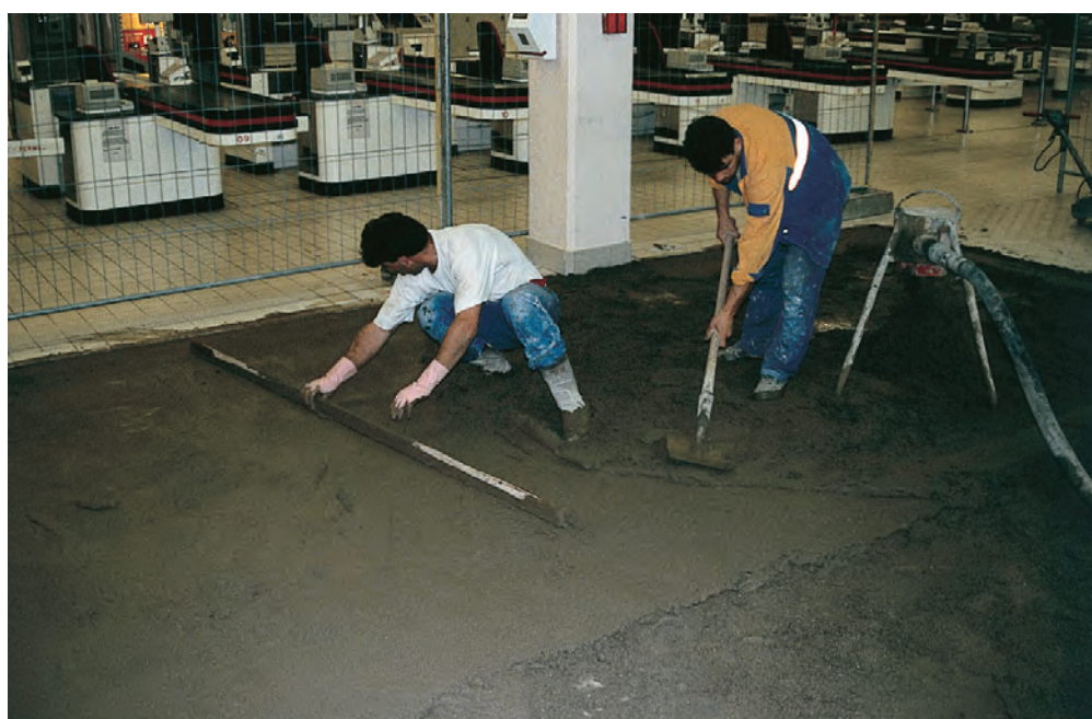
Fast repair of a screed in a supermarket
