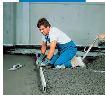
Using the straight-edge
