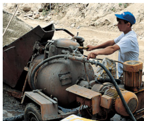
Mixing Mapecem with an automatic pumping unit
