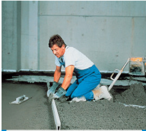
Using the straight-edge
