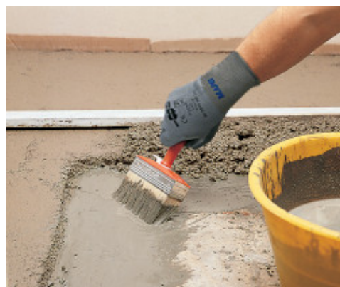
Spreading the anchoring slurry for bonded Mapecem screeds
