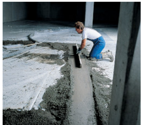
Preparing a levelling strip
