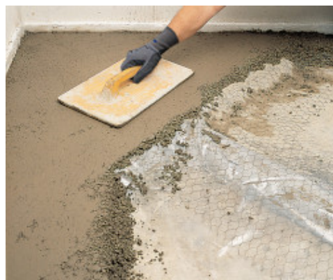
Covering pipes with Mapecem and reinforcement netting
