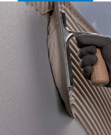
Installing floor covering using Ultramastic III
