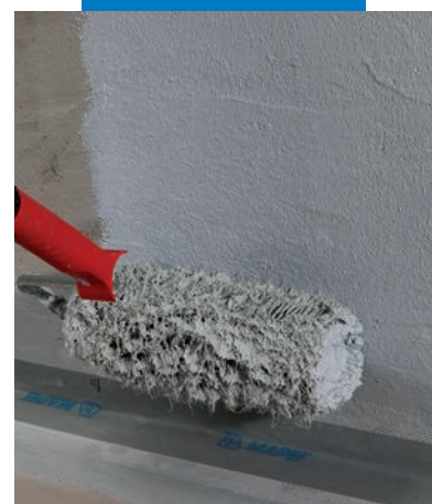
Application of Mapegum WPS with a roller
