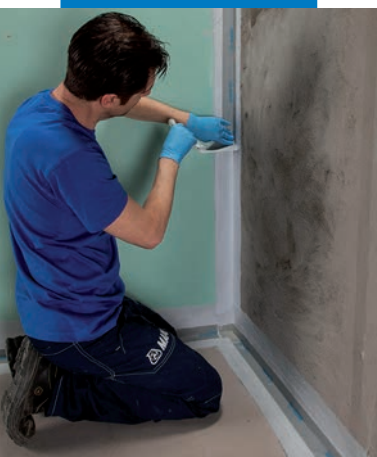
Application of Mapeband PE 120 using Mapegum WPS
