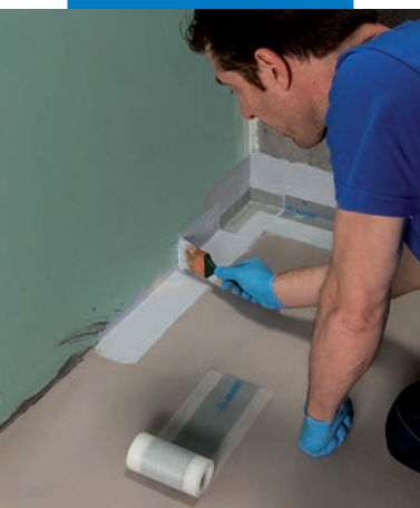
Application of Mapeband PE 120 using Mapegum WPS
