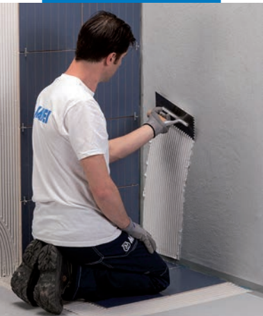
Installing wall covering using Keraflex Maxi S1
