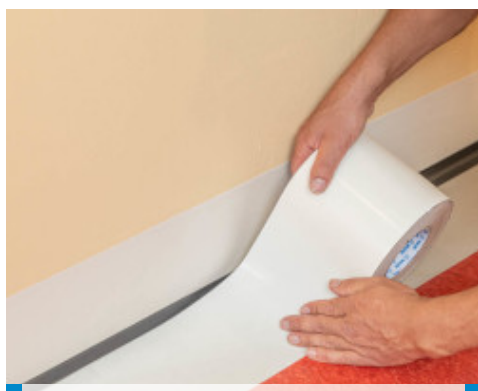
4. Placement of a new strip of Mapecontact Plus on the floor by overlapping the cove former slightly
