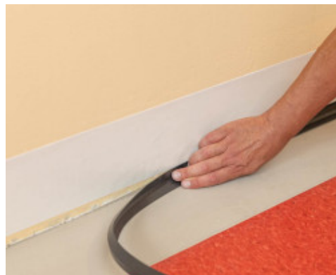
3. Installation of the cove former
