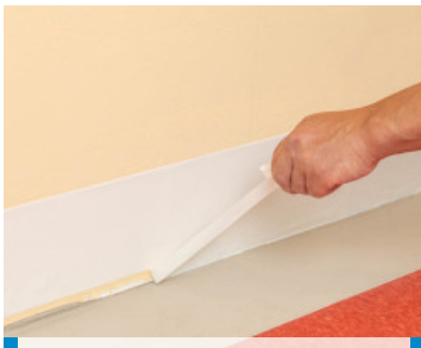
2. Removal of part of the protective layer of the dimensions of the cove former
