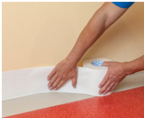
1. Placement of Mapecontact Plus on the wall
