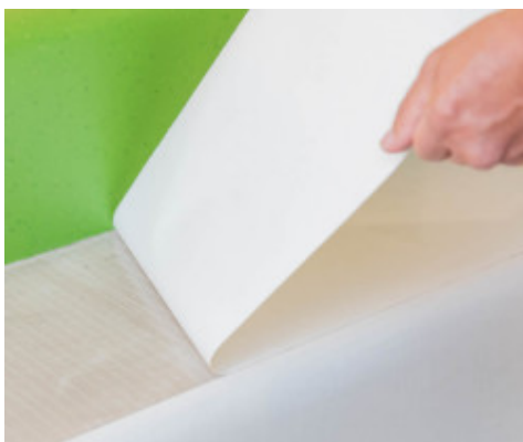
2. Removal of the protective layer from the tread and then from the riser
