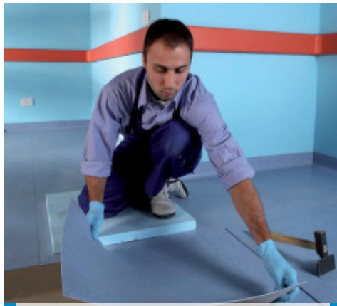
Installing PVC floor tiles
